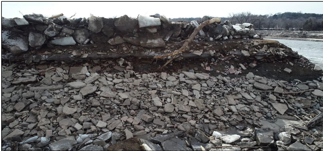
Figure 4.7 – Ice stacked on the north end of the south breach. The elevation of ice measured in the reservoir rim upstream from the powerhouse was about 4.5 feet above the design top of dam elevation (from NPPD video).
