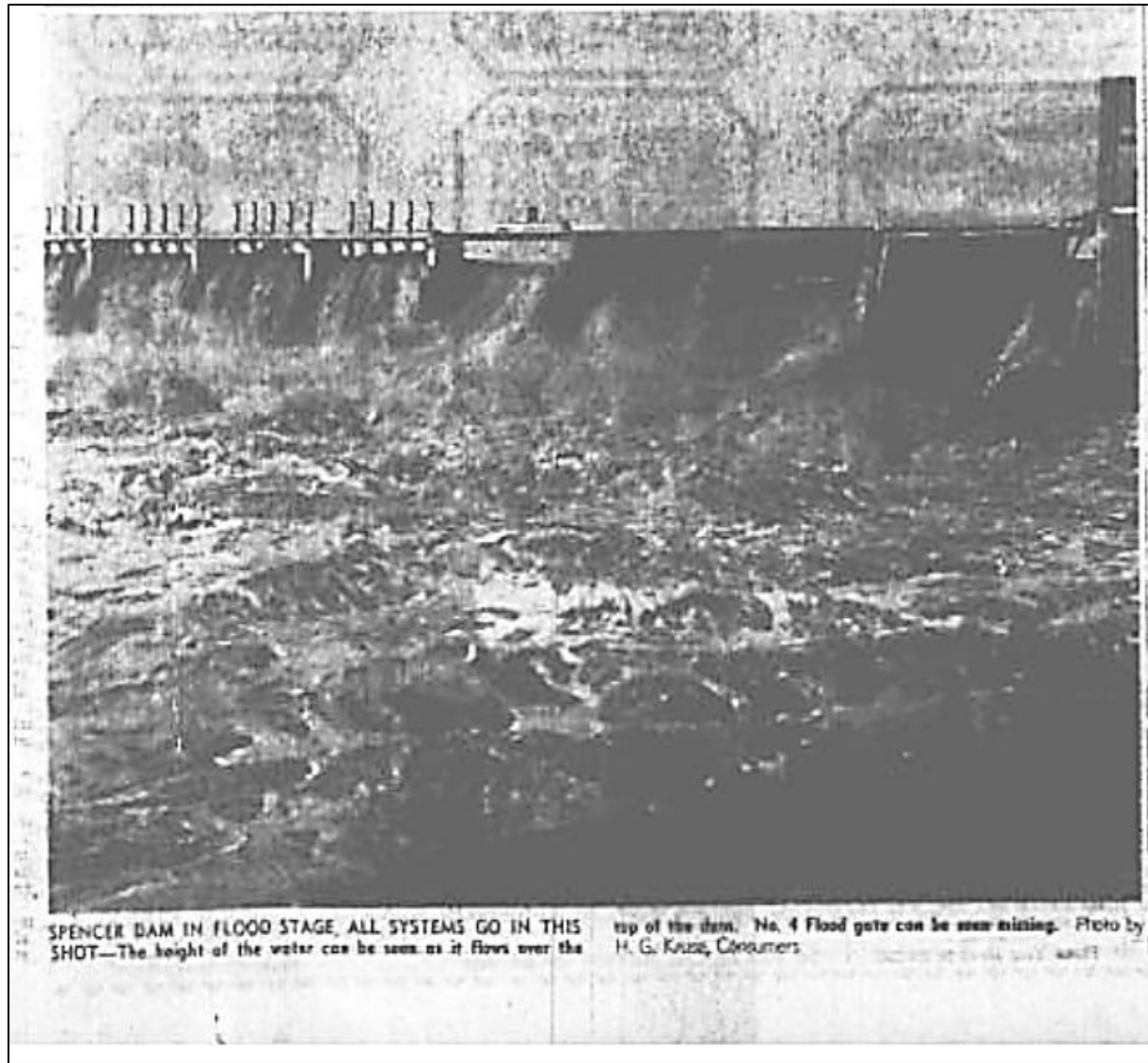
Figure 2.11 - Caption: "SPENCER DAM IN FLOOD STAGE, ALL SYSTEMS GO IN THIS SHOT" - The height of the water can be seen as it flows over the top of the dam. No. 4 flood gate can be seen missing. Photo credit Holt County Independent March 17, 1966, page 4. Research source: History Nebraska.
