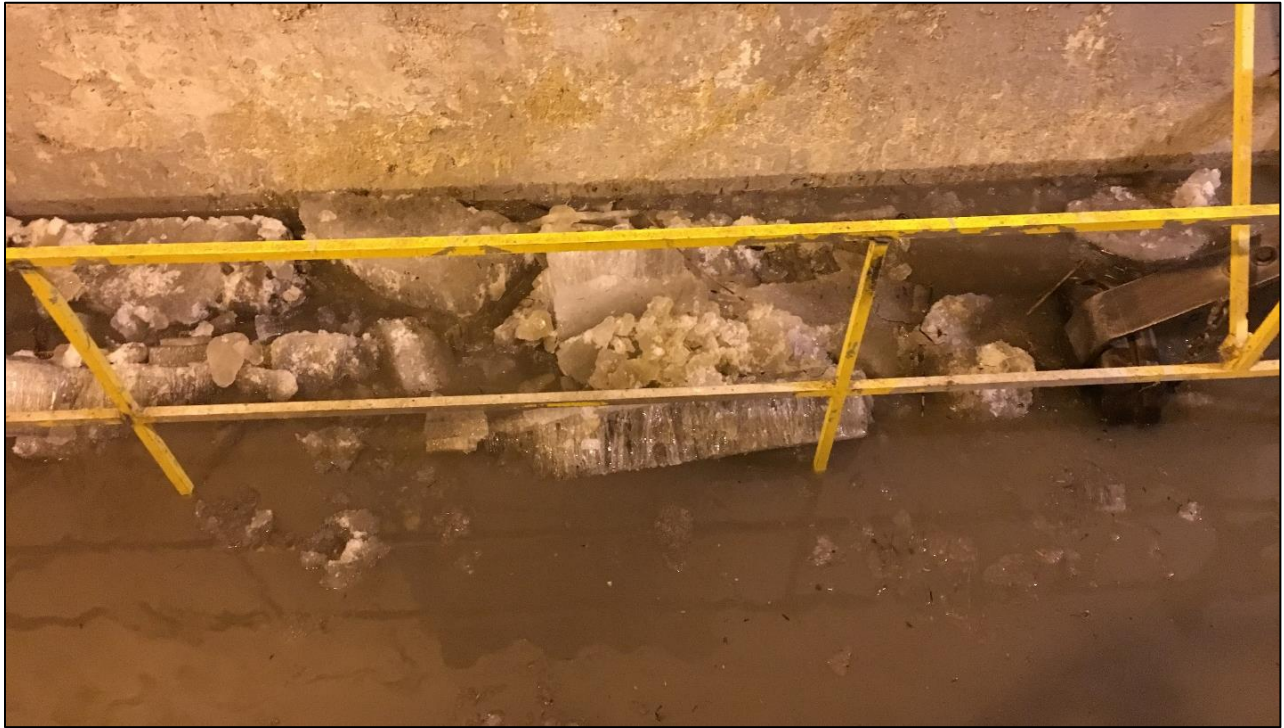
Figure 4.4 – Water and ice entering the trash-rake room at 4:38 AM on March 14. The trashrack slots are behind (upstream from) the railing (NPPD photo).
