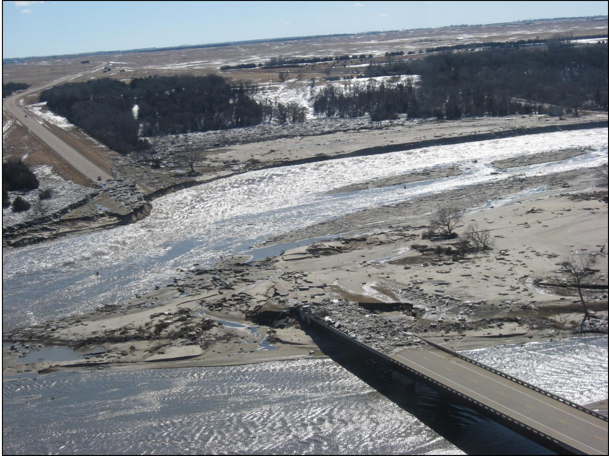
Figure 4.14 – View of washed-out Highway 281 approach ramp (looking south). Note the ice fields upstream and downstream from the road on the south bank (NPPD photo).
