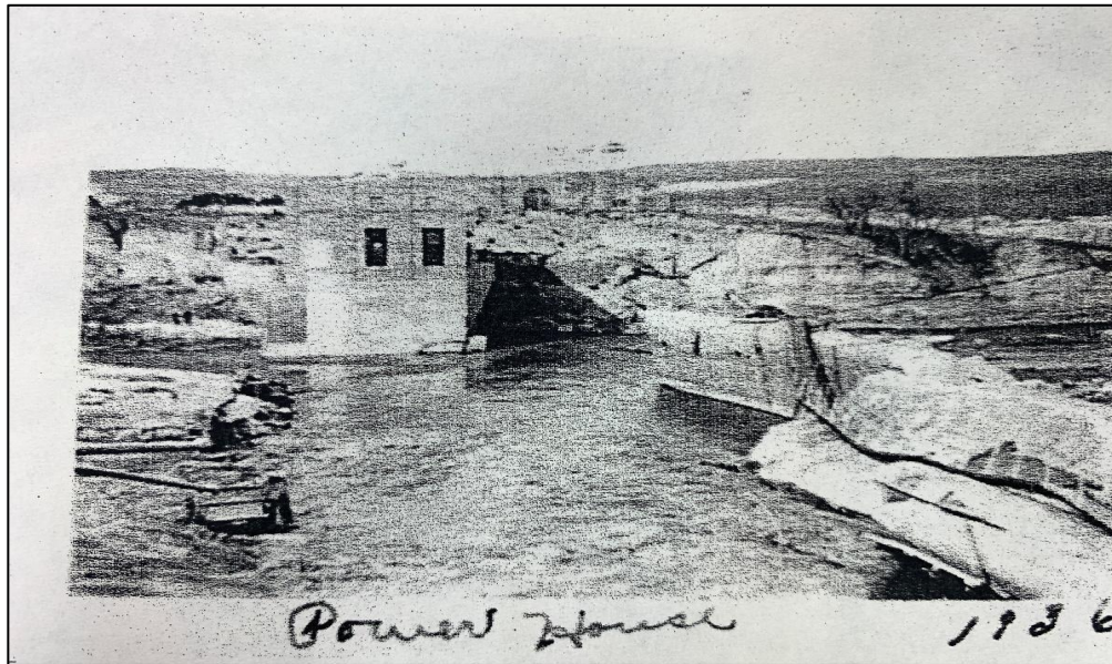
Figure 2.10 - 1936 Spencer Dam failure due to the concrete spillway sliding 50 feet downstream – NPPD photo.
